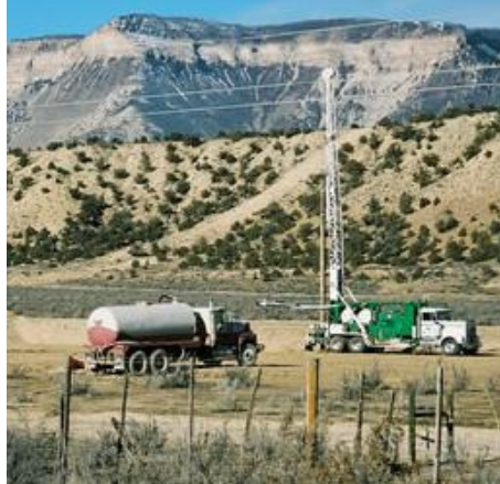
Photo of drilling site on the Roan Plateau (photo from BLM)
