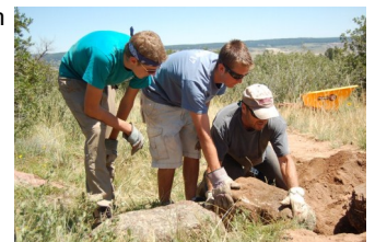
Zach Newton and his crew work on USFS Trail 715
